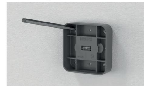
2b Drill holes with a diameter of 25mm using the marks made previously as guides
